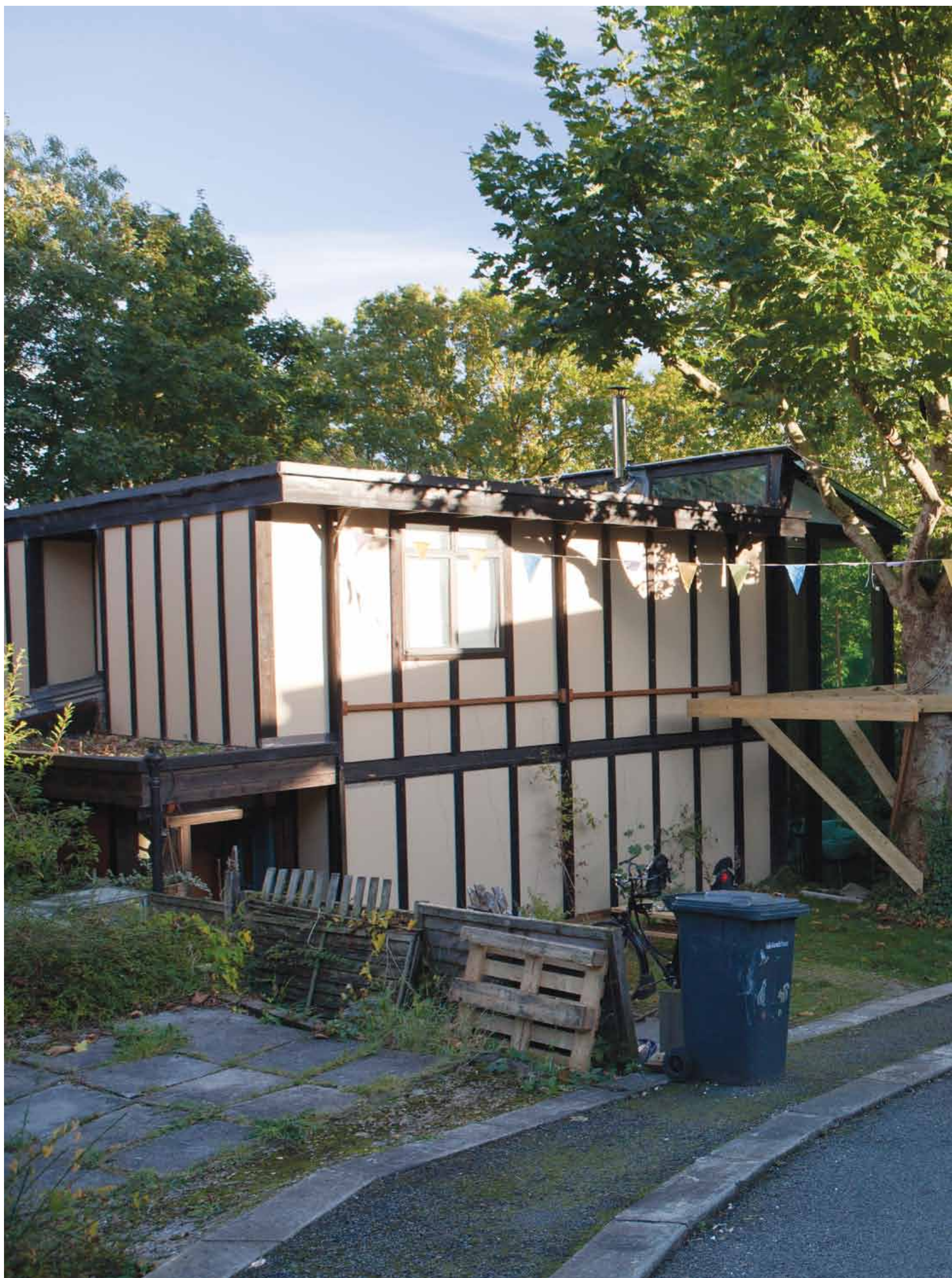
Walter Segal designed this simple self build system for small sites in Lewisham deemed unsuitable for council house building. The first phase of building started in 1979, the second in 1984. Altogether 50 homes were built in this way.
