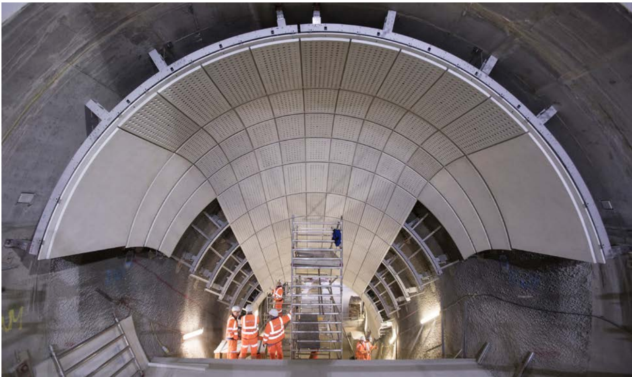
Game changer – glass-fibre reinforced concrete panels under construction at Bond Street’s Crossrail station
