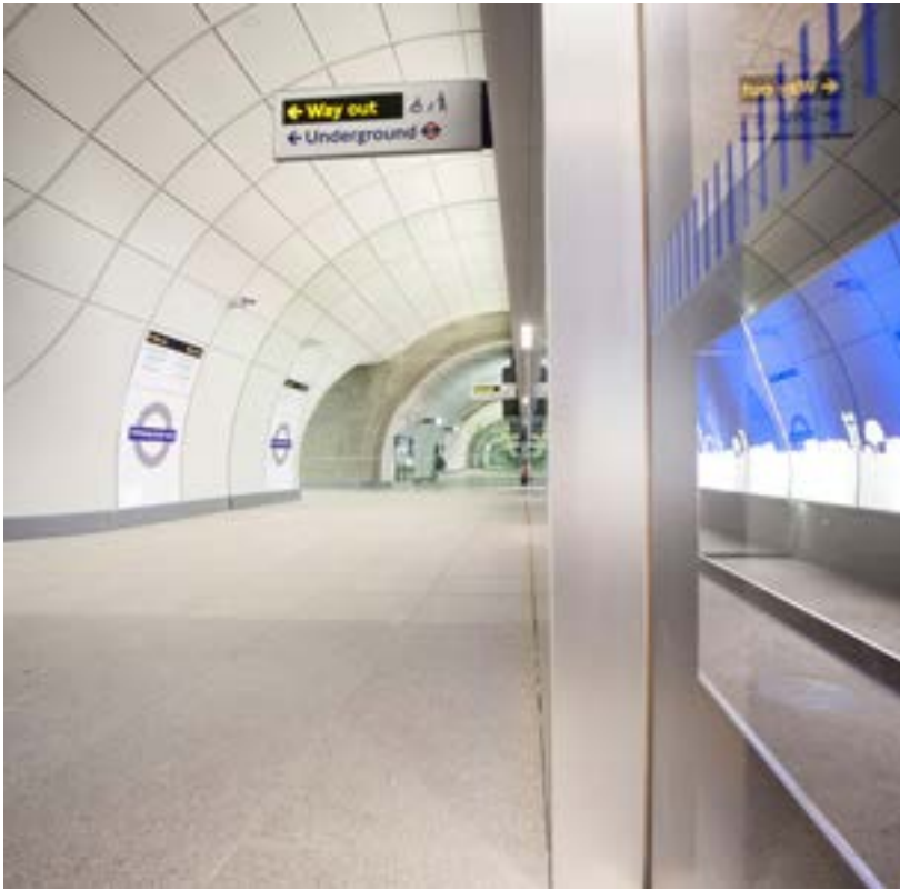
Wave-form: the cladding sits tightly against fluid-sprayed concrete forms
