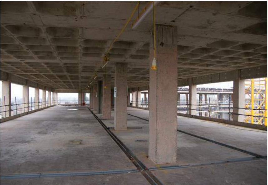
The original waffle slab floors
