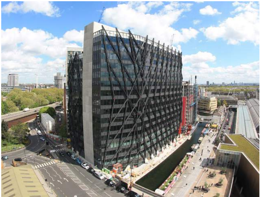
↓ The Fletcher Priest scheme features an external diagrid structure to free up the interior
