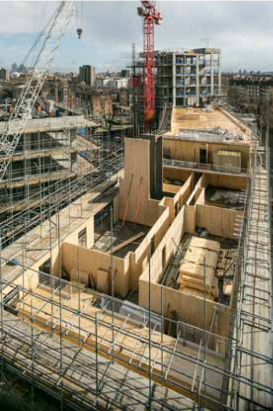
Engineered timber can quickly and safely produce sustainable developments
