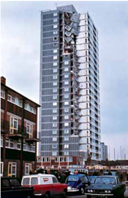
Ronan Point, West Ham, after building collapse
