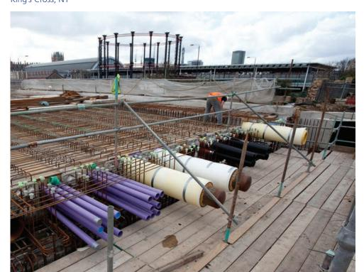
A site-wide network of pipes, cables and fibre optics has already been laid at King's Cross. Spare capacity is designed in from the start and empty ductwork will be available to future IT providers.
