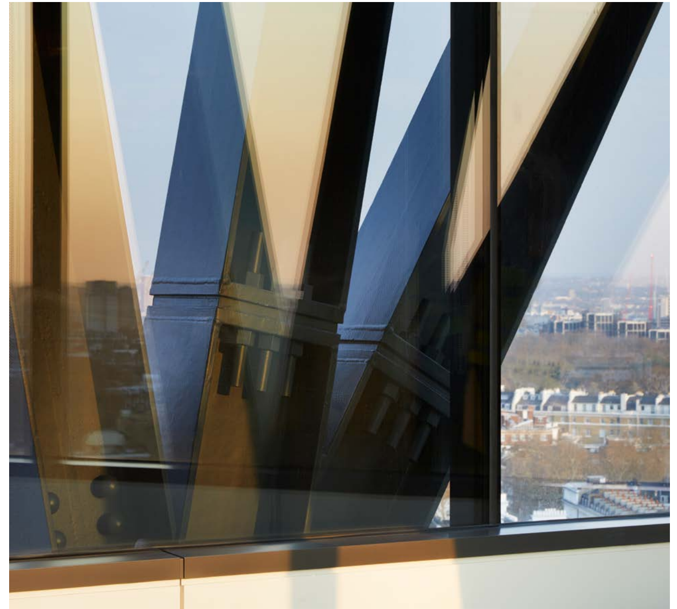
Dual purpose — an internal view of the exo-structure that provides partial shade to facades
