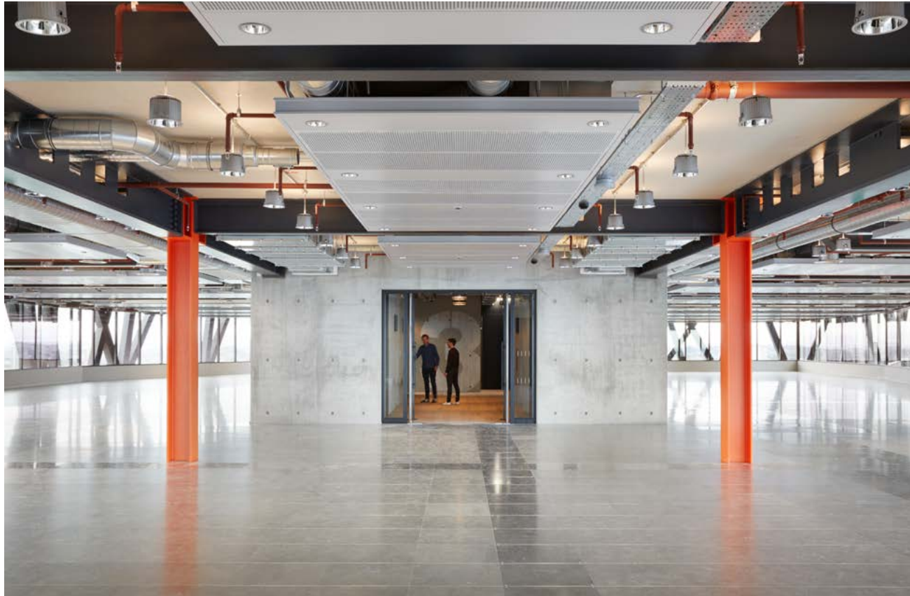
The Brunel Building's level 3 — the central core reduces, to be replaced by columns
