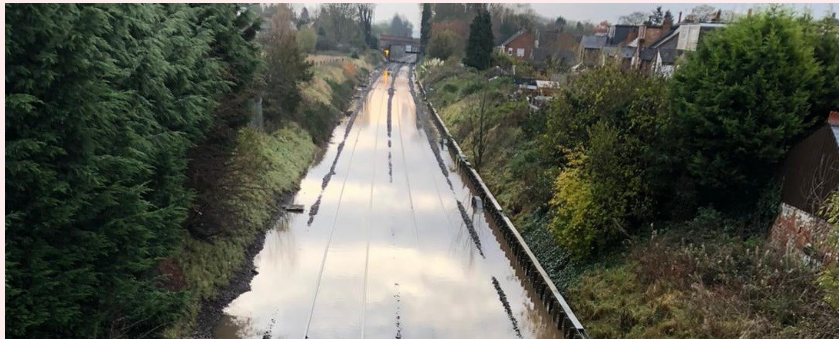
Top: biodiversity in rail | Bottom: flooded tracks
