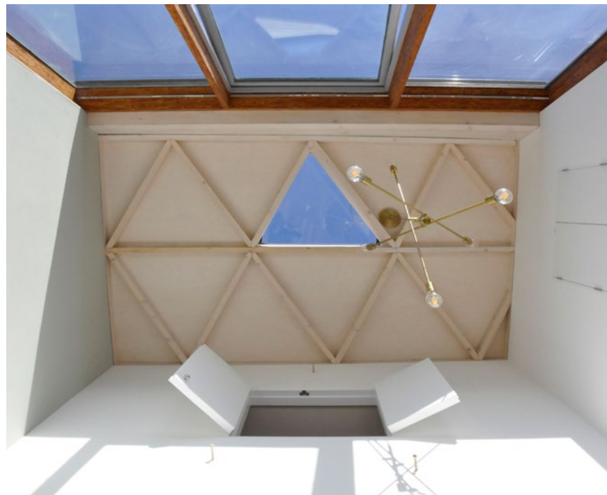
Section — the new lattice roof structure was raised to provide additional bedroom space
