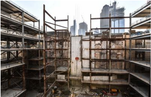
Steel frame demolition
