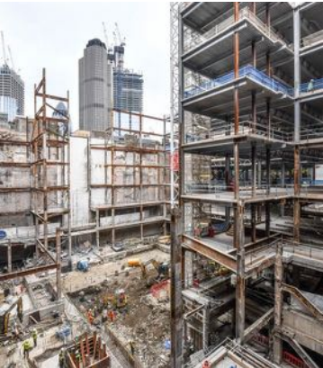
Steel frame demolition
