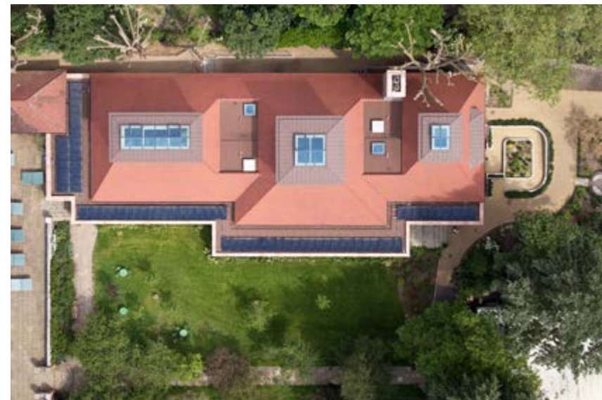
Photovoltaic panels on the roof helped achieve a BREEAM 'excellent' rating
