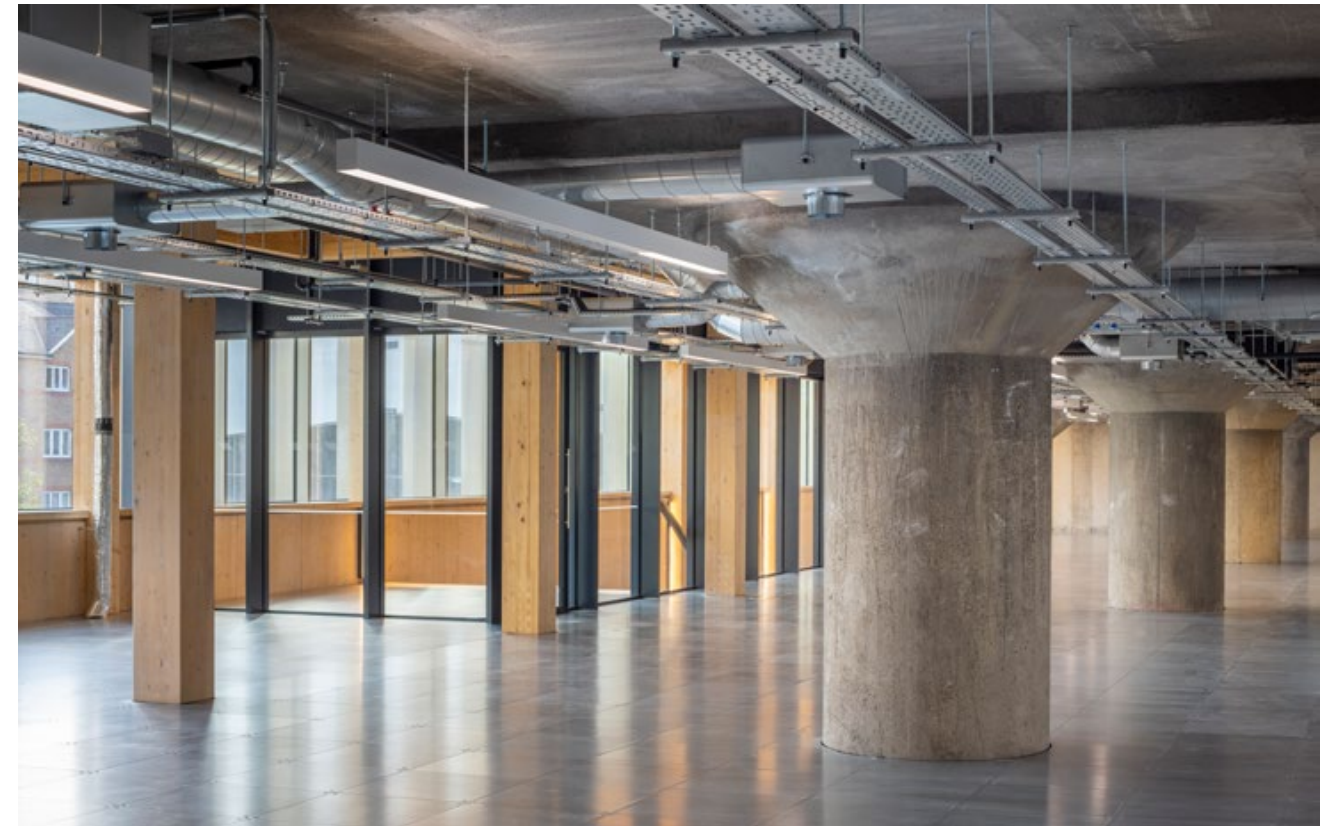
The original structure features columns over a metre in diameter
