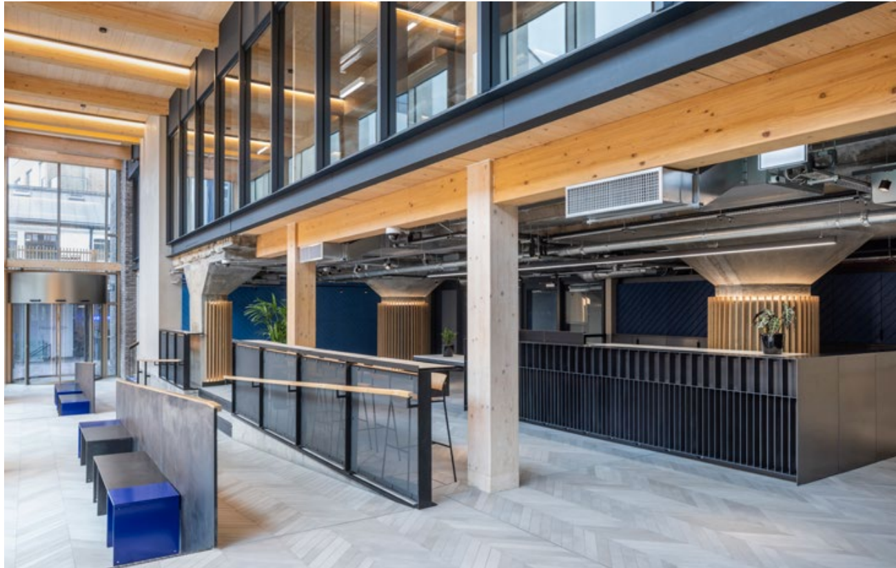
The building retains the existing structure — some 655 tonnes of embedded carbon
