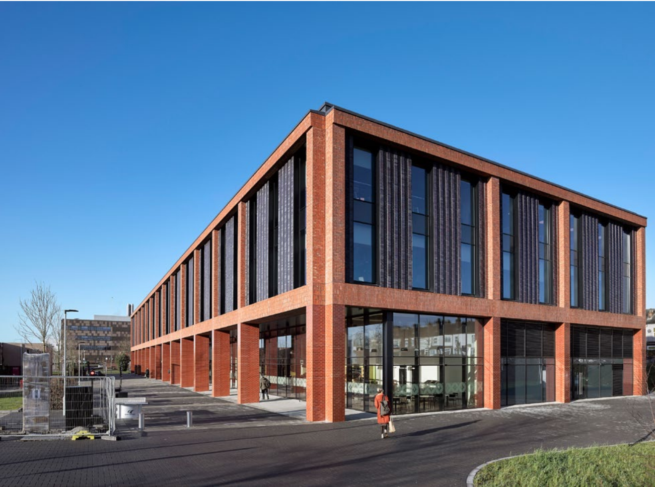
Staffordshire University’s Catalyst Building in Stoke-on-Trent, whose colonnade provides shading in summer but allows solar gain in winter
