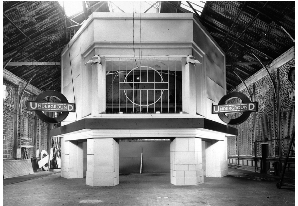
Model railway — a full scale timber and paper mockup of the proposed Northern Line Stations design concept, 1925
