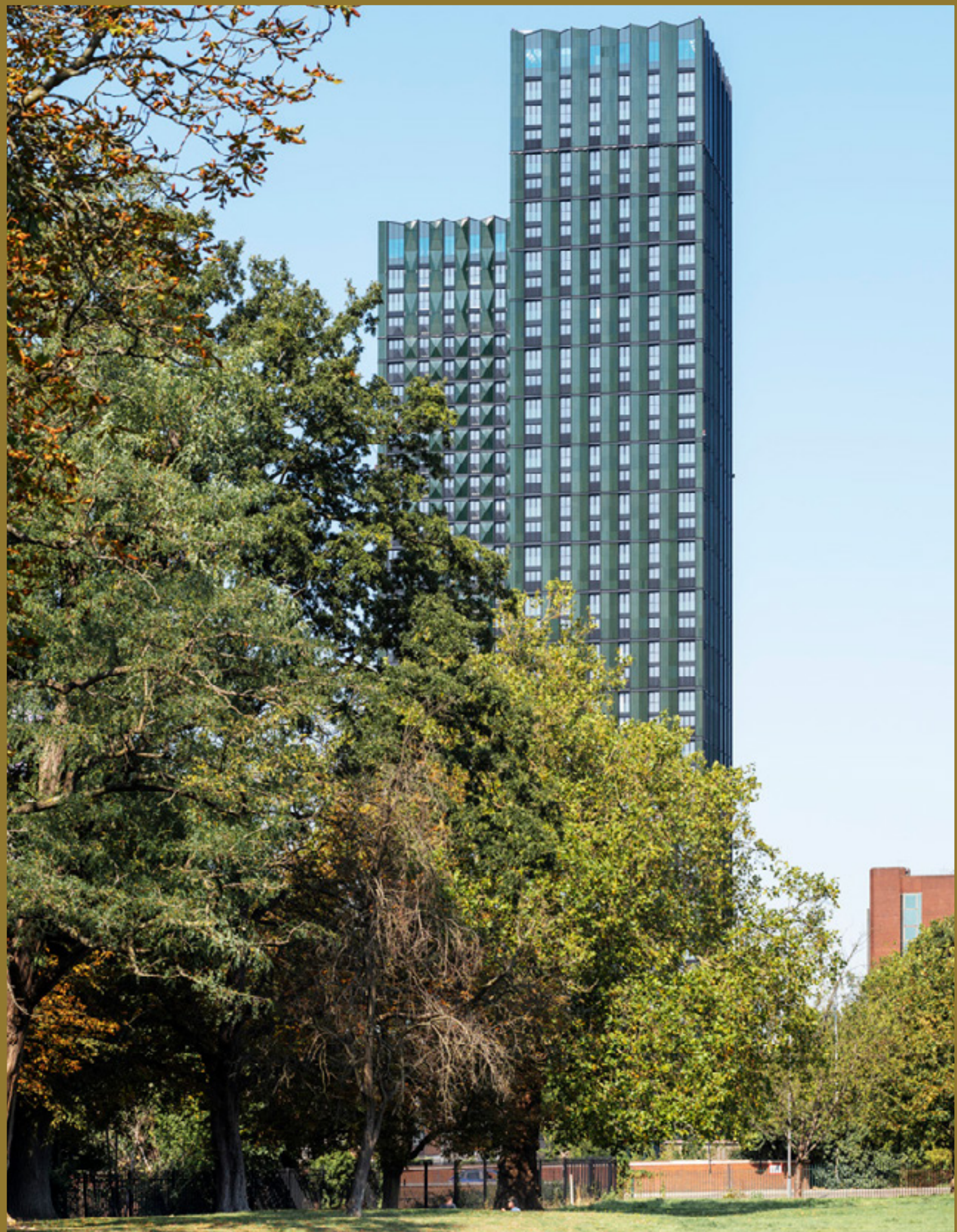
Ten Degrees in the LB Croydon by HTA and Tide Construction is the world’s tallest modular building delivered in just 26 months using modern methods of construction, completed in 2020.
