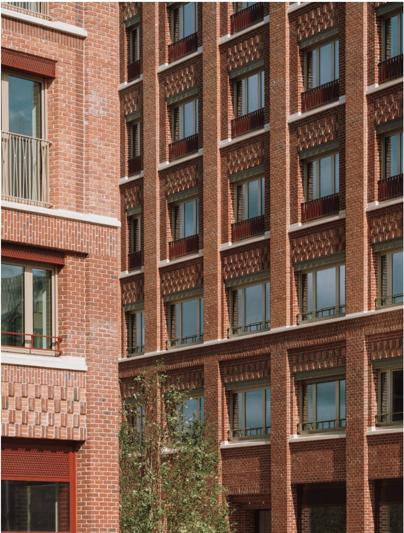
Shading it—a distinctive feature of the scheme is the 500 external solar-control shutters
