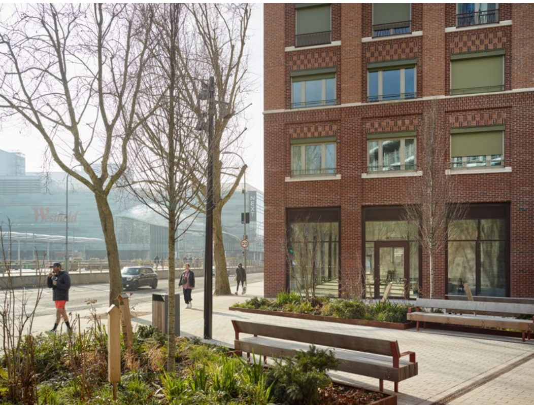
MacFarlane Place — the scheme comprises 143 affordable-tenure homes
