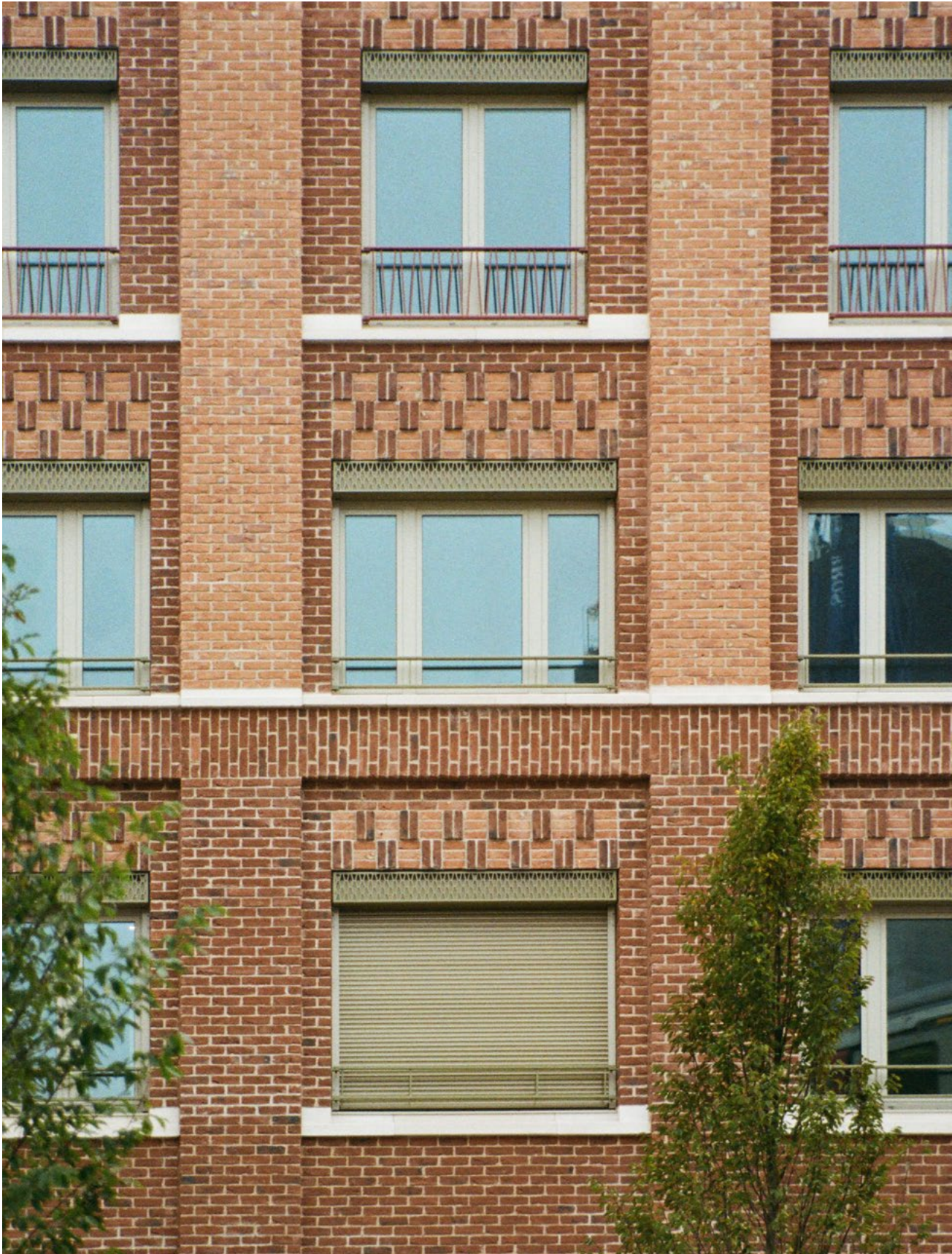
Shutters allow residents to shut out all unwanted solar gain when they're out, allowing them to return to a cool, comfortable home
