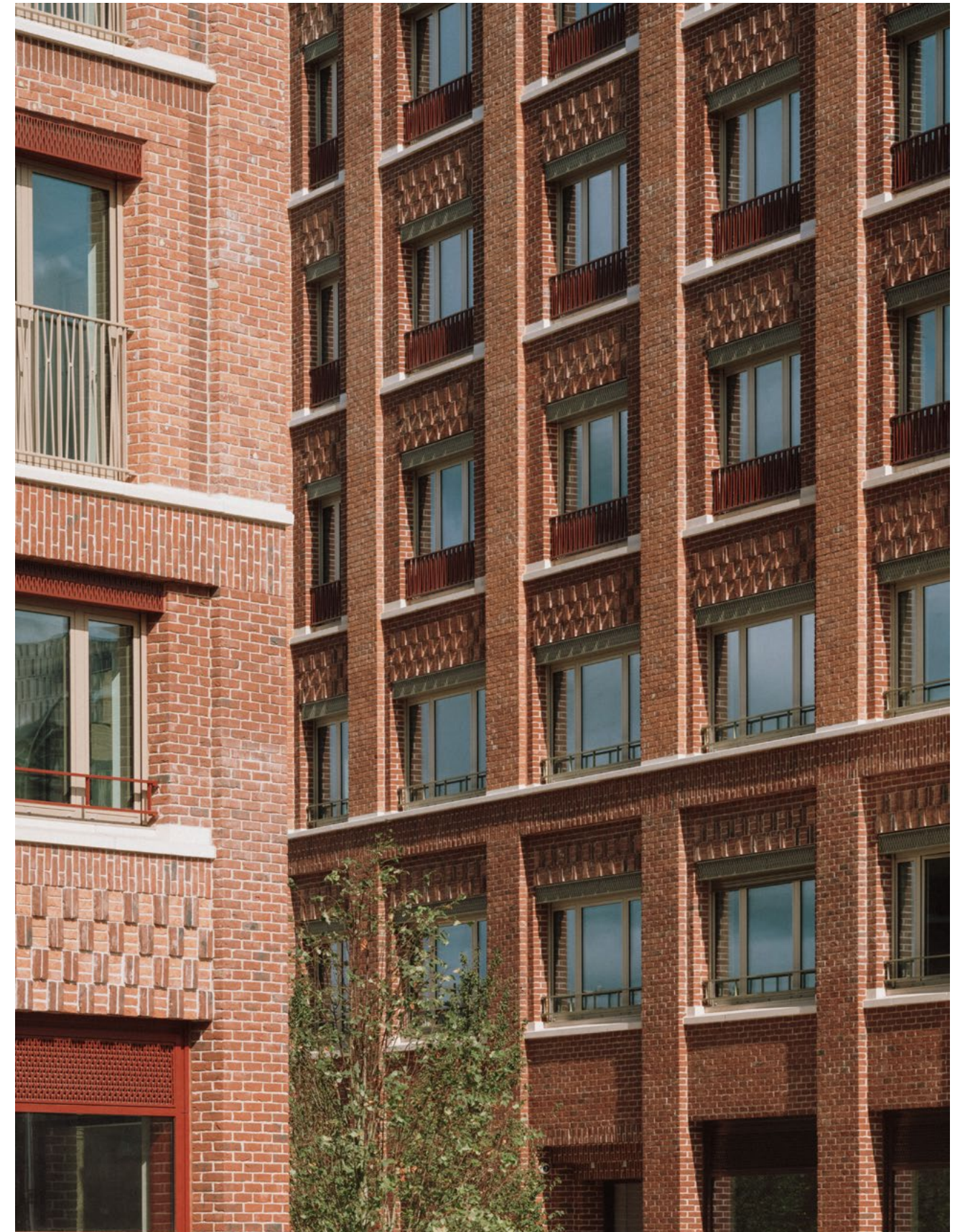
Shading it—a distinctive feature of the scheme is the 500 external solar-control shutters
