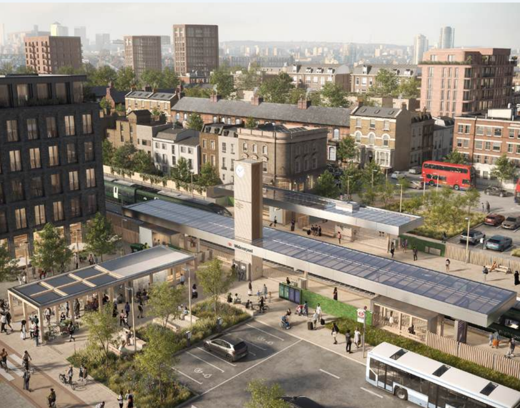
Network Rail HubStation Standard Station Design with integral upgradable PV panels. © Network Rail/7N Architects/Pillar Visuals
