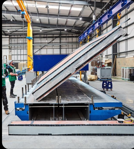
Advanced offsite fabrication
